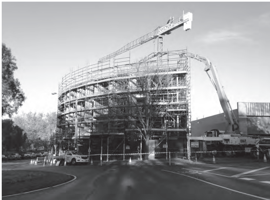
Construction at 1 Shiel Street is well advanced
