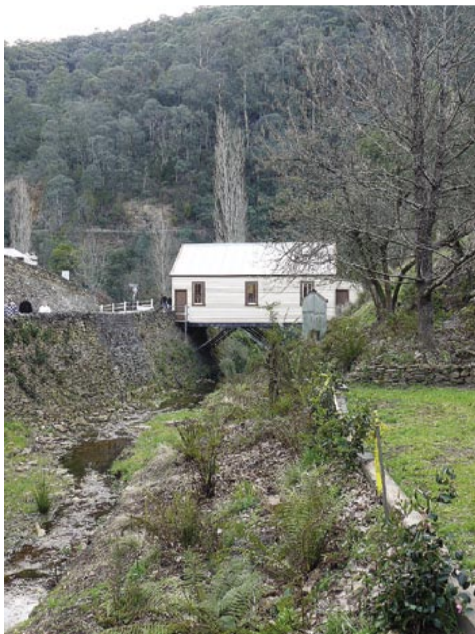
The old fire station straddling Stringers Creek
